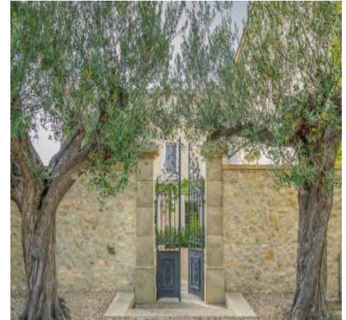
Gates to courtyard
